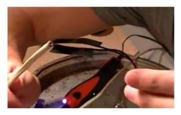
Once your done adding all the sensors to the cords, move the heat shrink wrap into place and heat it with a lighter until it securely seals the new cord.
