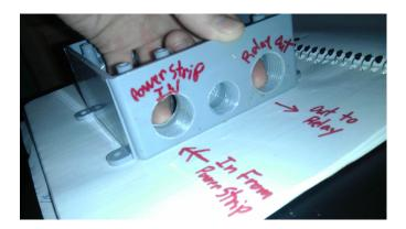
Insert and screw in the cable connectors.
