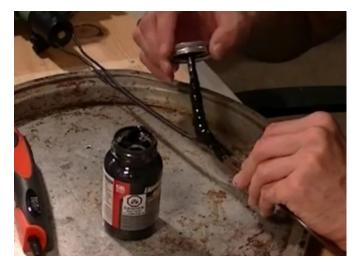
So far we have soldered the two wires, wrapped them with electrical tape, and added water proof liquid electrical tape as moisture sealant. Finally, before the liquid electrical tape dries, we will slide the heat shrink tubing over the solder point and secure it by running a flame over it.
