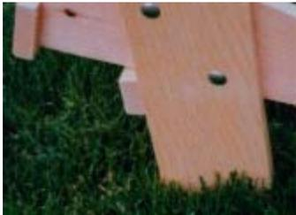
**2** - Cut part **S1**, the front joiner strip, to **1 3/4" x 52 5/8"** (4.5cm x 133.5cm). Plane the edges, sand and attach with one screw into the 4 front legs D. Drill pilot holes for the outside screws, since they will be close to the ends. Be sure that the ends of S1 are flush with outside edges of the front legs, and tight to the **undersides** of sides A, as shown.
