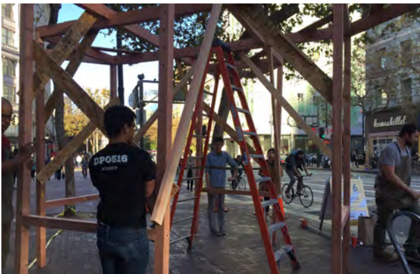
7. Secure Frame 1 and Frame 2 into The Notches; Remove Temporary Supports
