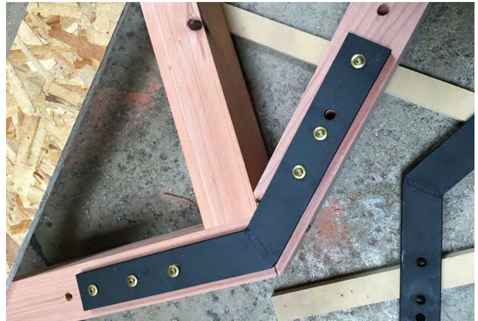
Attach Metal Reinforcements to Top of Arbor Frame
