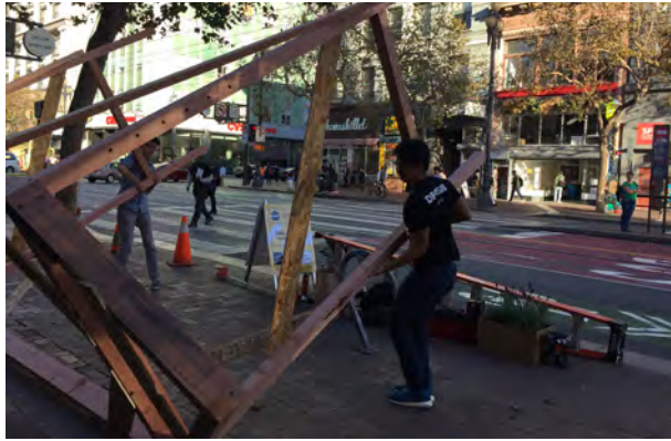
2. Rotate Assembled Frame 2 to the side
