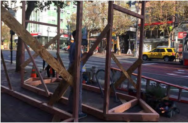
1. Attach Posts to Arbor Frame 2 First with 10# Lag Screws
