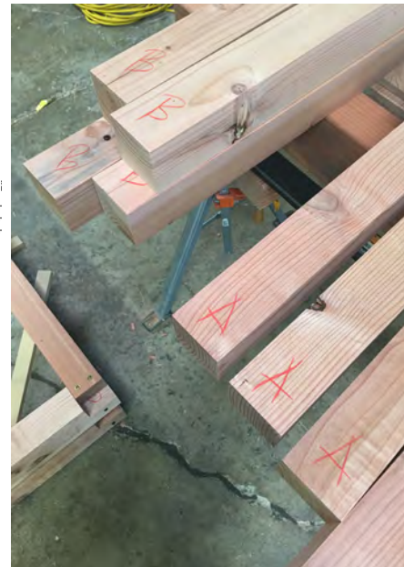
Marking and Preparing C and D Members for Cutting
